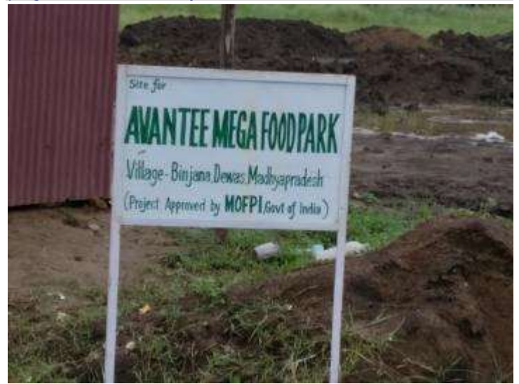
Exhibit 67. Mega Food Park – Dewas, MP – Construction work in progress, could take few years to scale
