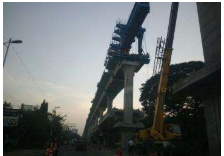
Exhibit 91. Metro construction - Nagpur metro work in full swing
