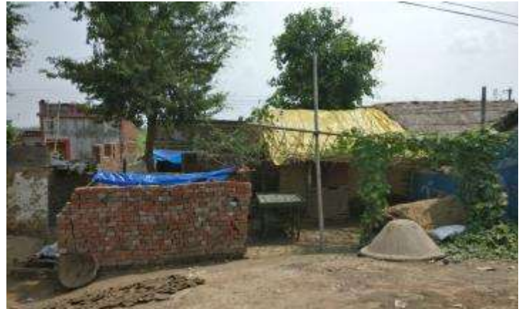
Exhibit 89. Bihar, similar to UP, sand mining restrictions had halted the construction work during past two months
