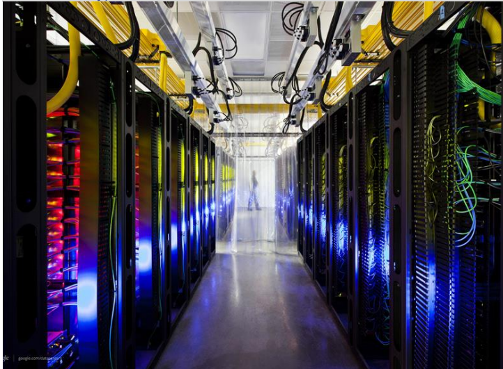
Exhibit 17. Inside a typical data centre rows of high density server racks are arranged... Interior of a typical data centre
